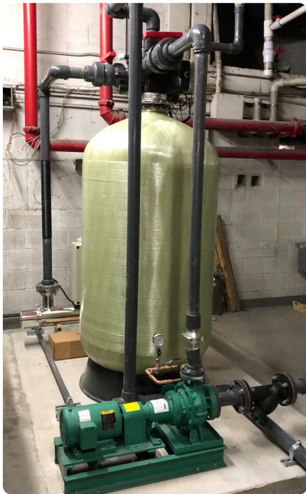
EasyWater SedimentShield Filtration for CTF-100
