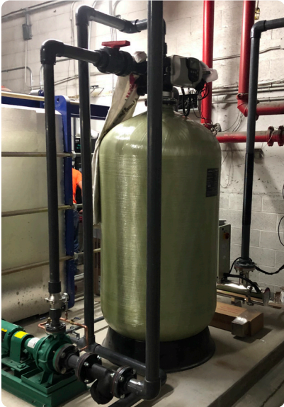
EasyWater CTF System: Model CTF-100 Installation at CocoWalk
