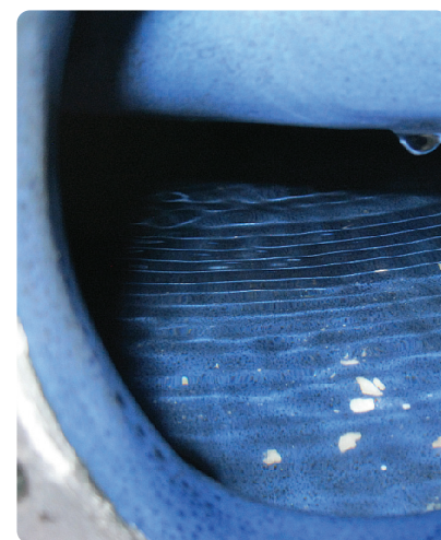
AFTER: 4 Months — Water Heater with EasyWater Treatment
