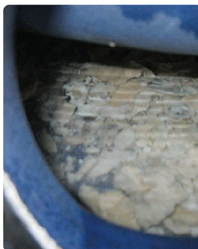
BEFORE: 4 Months — Water Heater without EasyWater Treatment
