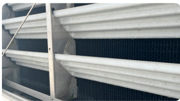
Even with open louvers the BAC cooling tower fill is clean and free of algae, biofilm and scale
