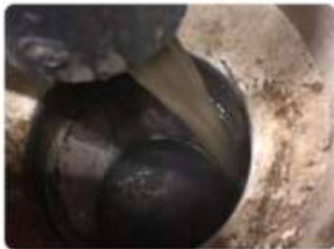
Dirt and debris being removed during backwashing
