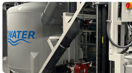
SedimentShield backwashing filtration tank
