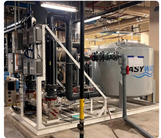
EasyWater Cooling Tower Treatment System Model CTF-500-S installed
