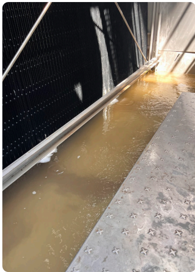
Inside one of the cooling tower basins before the CTF System was turned on (See after photos on page 2)
