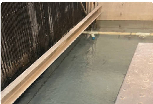
Cooling tower basin 1 year after CTF System was online
