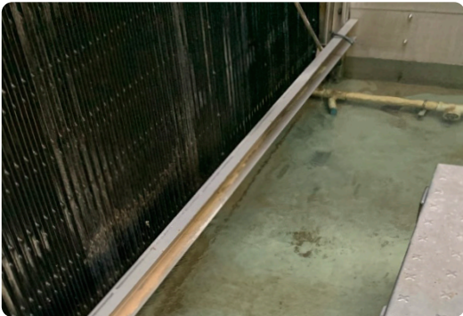
Cooling tower basin 2 weeks after CTF System was online
