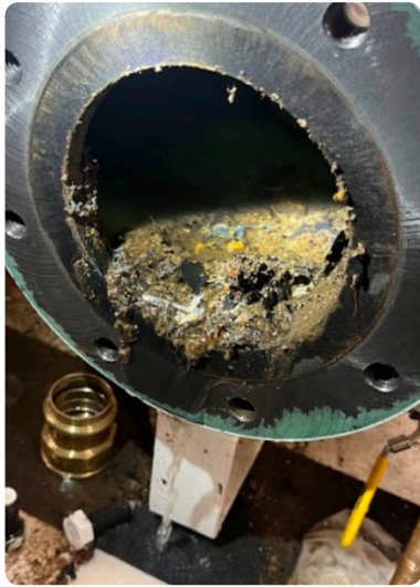
Cooling tower debris being removed during startup
