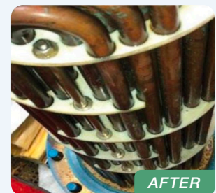
Example of domestic heat exchanger after 6 mo of scale removal & prevention treatment
