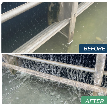
Improved sump water clarity after two weeks of CTF System operation
