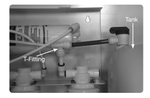
Connect black <sup>3</sup>/<sub>6</sub>" line from permeate pump output to <sup>3</sup>/<sub>6</sub>" fitting drain saddle.
